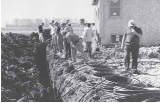
A horizontal loop being installed.
